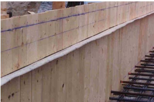
The split form should firmly hold the waterstop in position to prevent misalignment of the waterstop during concrete placement. A tight fit is also necessary to prevent excessive leakage of concrete paste, which could lead to honeycombing of the concrete.
