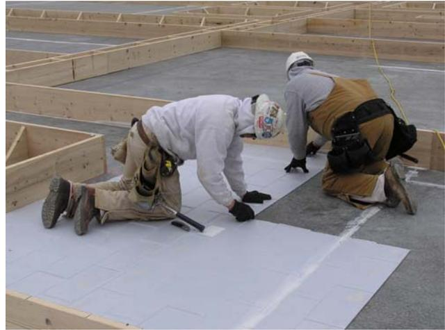
The concrete and the form liner must be clean and dry during installation. After initial installation, keep the concrete surface dry, as moisture between the plastic and the concrete can break the adhesive bond. Sealing at the form liner joints will aid in maintaining this bond.
